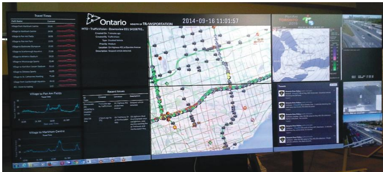
Dashboard display in MTO Downsview TOC showing travel times, the latest unplanned issues, and nearby traffic cameras. Formatted for a large 3x2 1080p display wall
